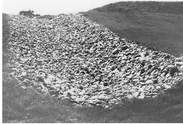
Figure 4—The field chute with D<sub>50</sub> = 188 mm (0.617 ft) and S = 16.7%.
