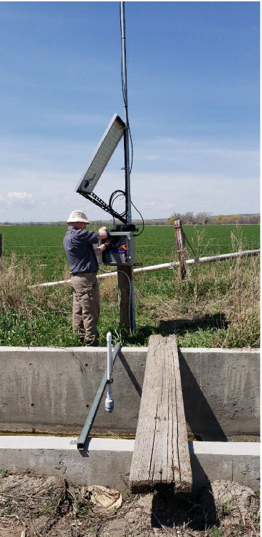
Solid support across cement channel
