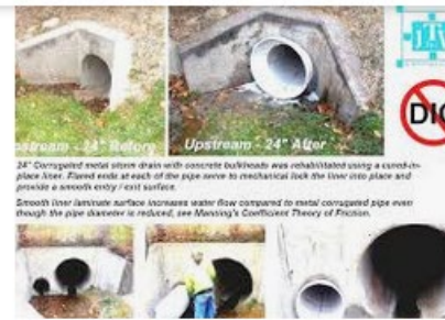
Cured-in-place Pipe - Water Pipe Lining manualrecords.blogspot.com
