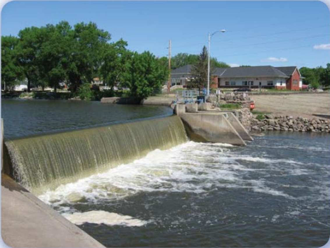
Upstream view of dam from right bank
