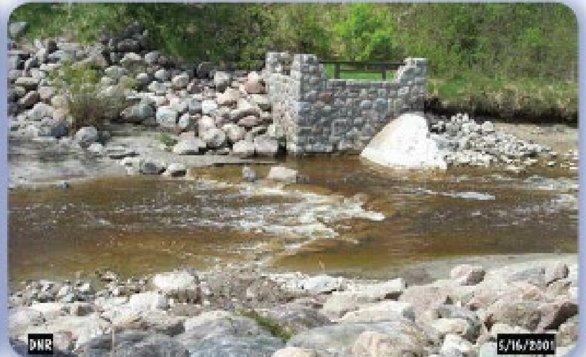
Upstream view of removed dam and constructed boulder weir
